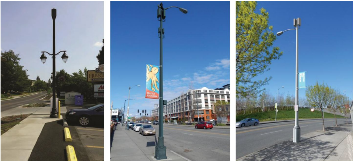
Examples of a well-designed small cell facility
