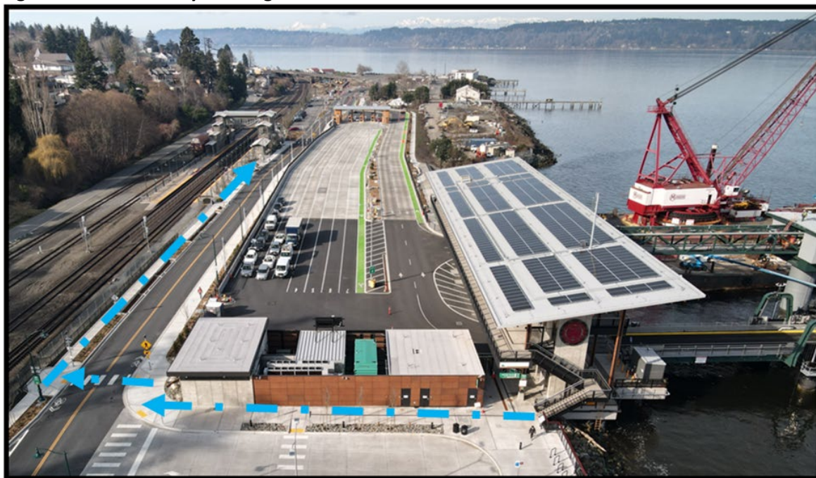
Figure 2. WSDOT Ferry Passenger Pedestrian Connection to Mukilteo Sounder Station.
