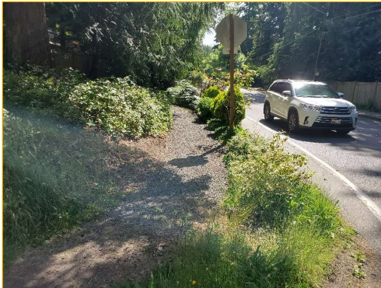
Photo E.2 – Facing north from the east side of 53 rd Ave W. Runoff travelling south enters a catch basin and is conveyed west through the existing tightlined storm system.
