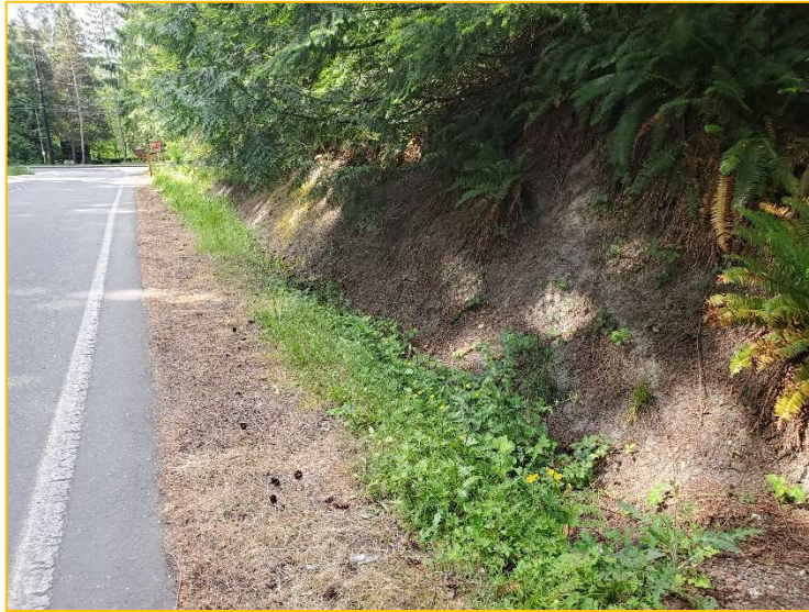
Photo E.1 – Facing south from the eastern property edge. Runoff enters drainage swale adjacent to the west side of 53 rd Ave W and is conveyed south.
