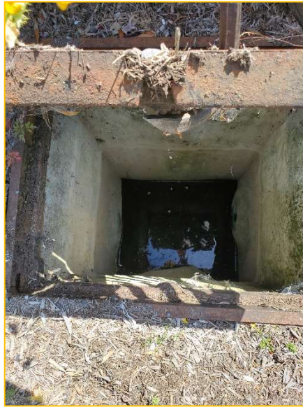
Photo W.5 – Facing east from the east side of Hargreaves Pl. Runoff enters existing catch basin and travels west across Hargreaves Pl.
