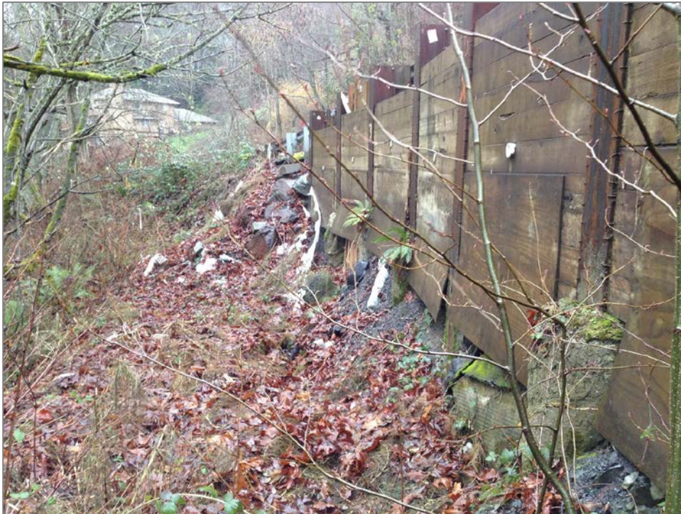
Photo 6. Failing portion of retaining wall, and area of wetland buffer that will be temporarily affected.
