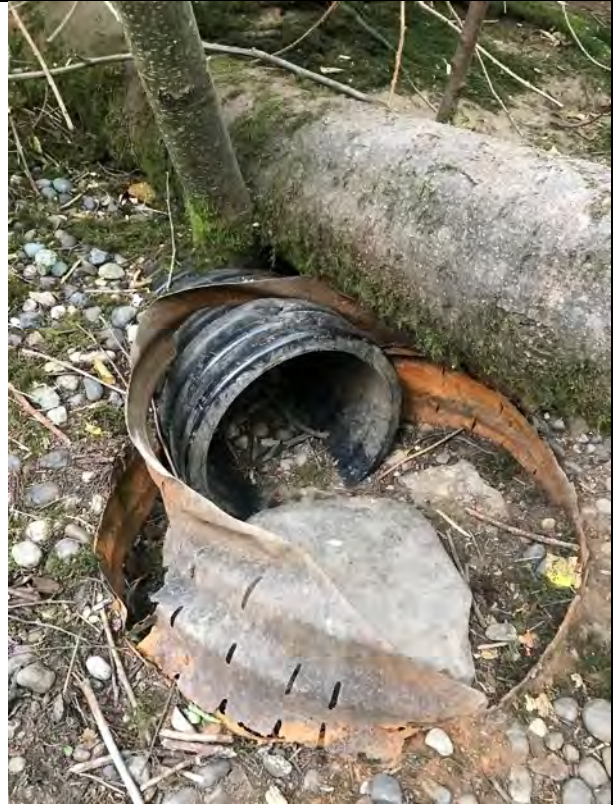
Photo 2: Existing stormwater pond outlet culvert. Photo taken October 2020.
