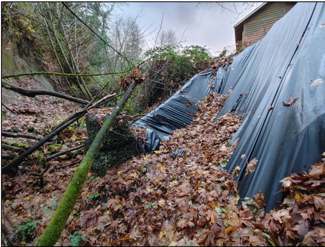
Figure 1 Hillslope failure/Project Area, covered with plastic sheeting as temporary erosion control.
