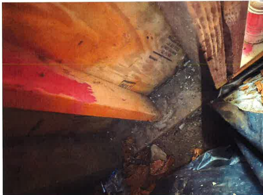
Figure 2: Cripple Wall studs and Sill Plate to the Concrete footing
