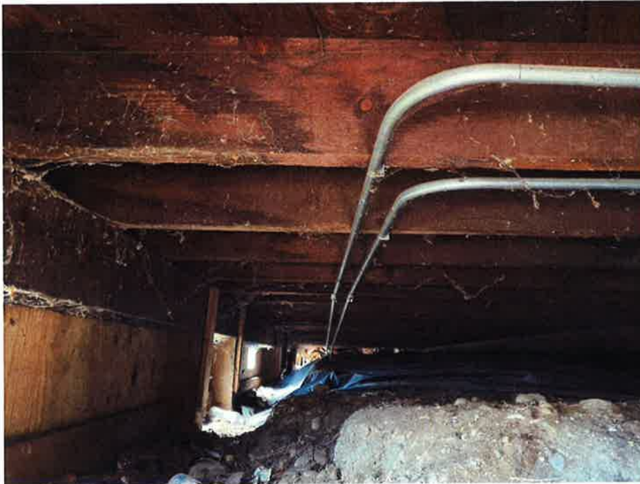
Figure 5: Lower level floor joists with floor beams
