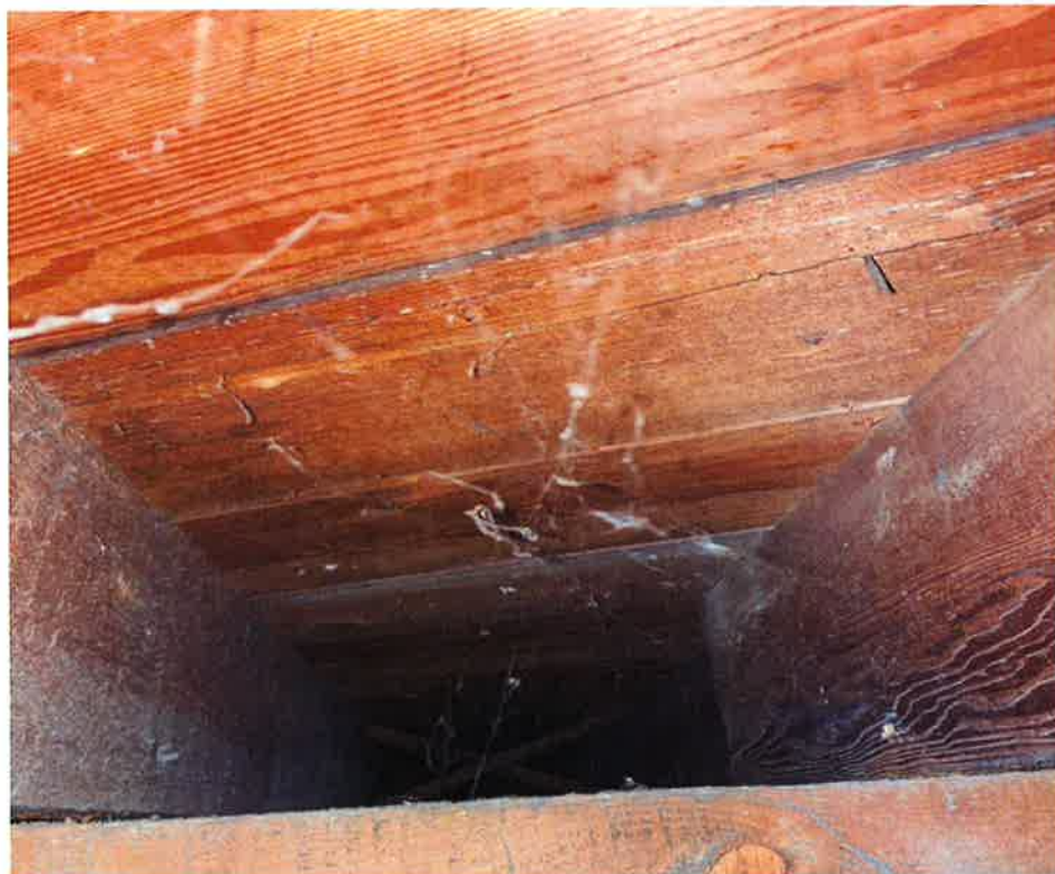
Figure 6: Floor Sheathing – 1x decking
