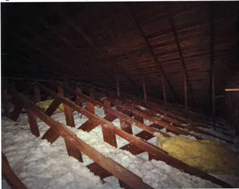
Figure 11: Roof Framing – Truss A w/ Over framing & vertical supports
