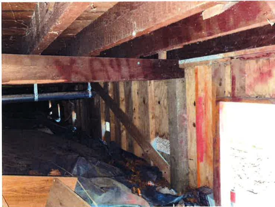
Figure 4: Cripple wall between footings and lower level floor framing
