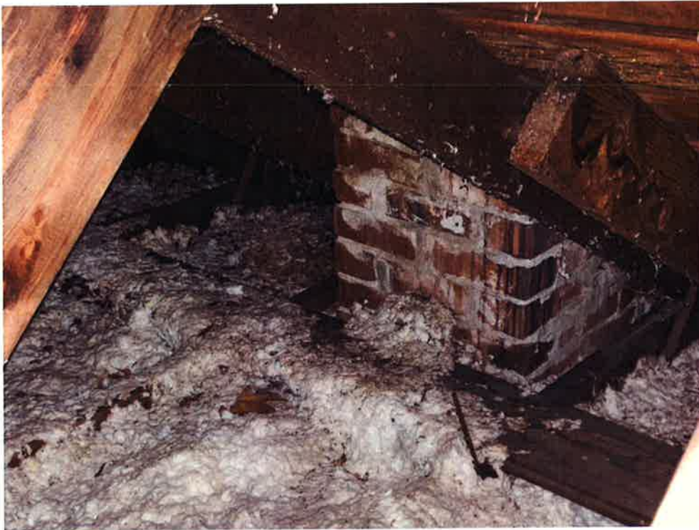
Figure 17: Chimney – No lateral bracing
