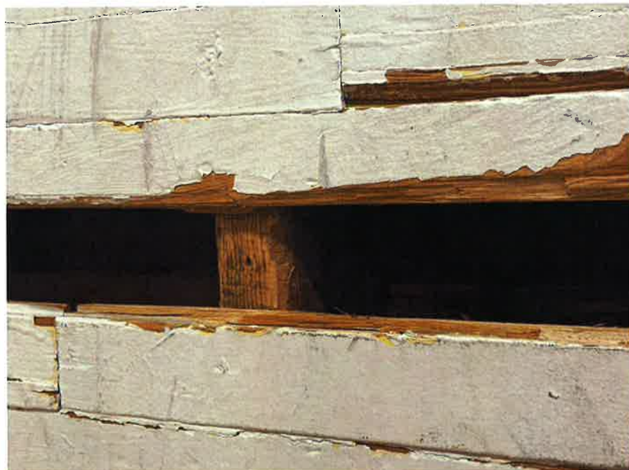
Figure 8: Wall Studs w/ Interior 1x decking
