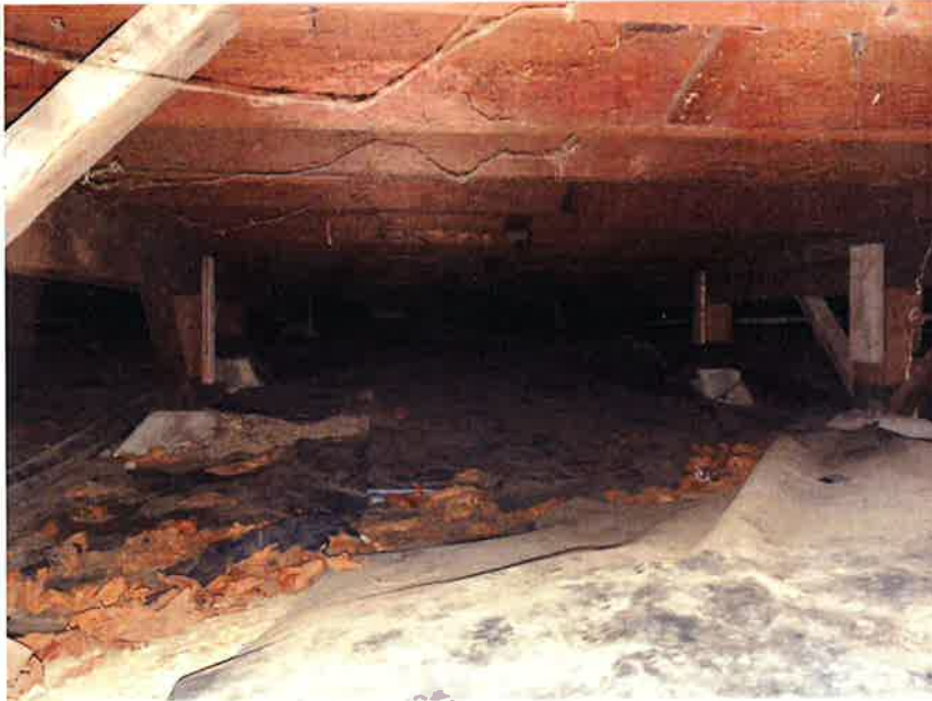
Figure 1: Intermittent Concrete footings w/6x6 Posts
