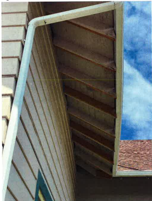
Figure 16: Roof Framing – Rafter Tails Failure and Sistered with new ones
