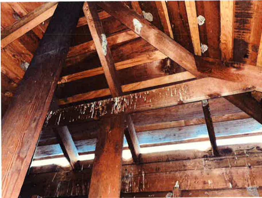
Figure 15: Roof Framing – Truss C Dutch Gable End
