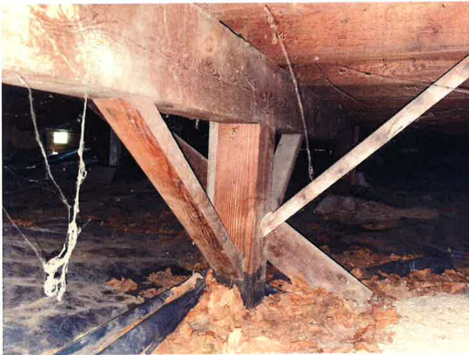
Figure 3: Intermittent post footing w/ kicker supports
