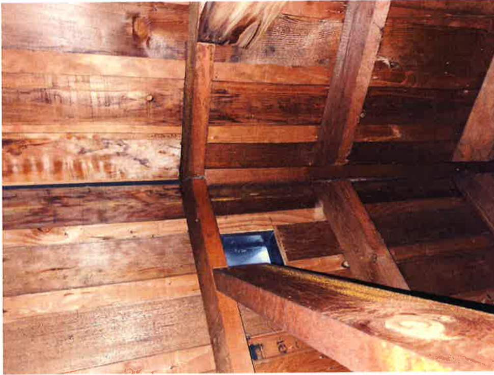
Figure 10: Roof Sheathing – 1x decking under 1/2" plywood.
