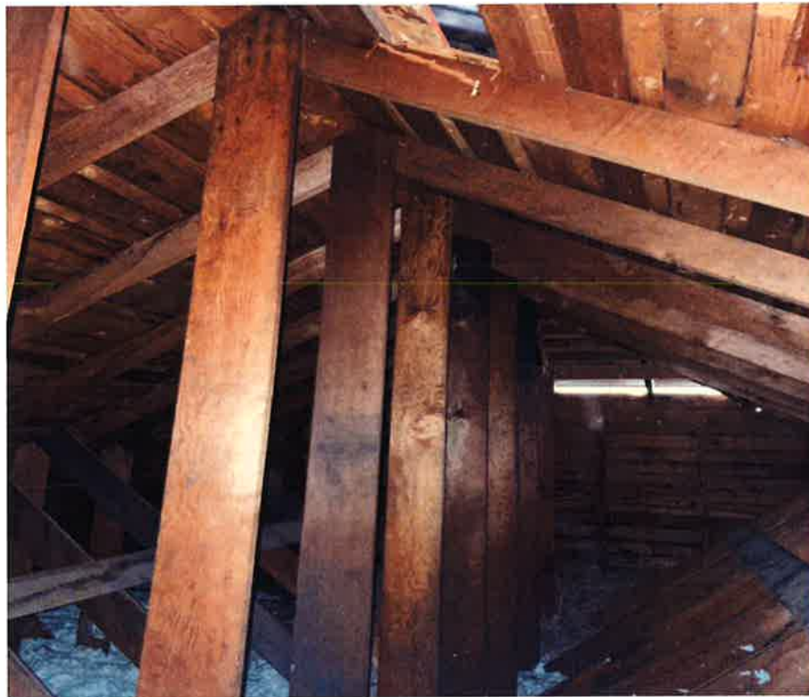
Figure 15: Roof Framing – Truss C w/ 1x10 Web Members
