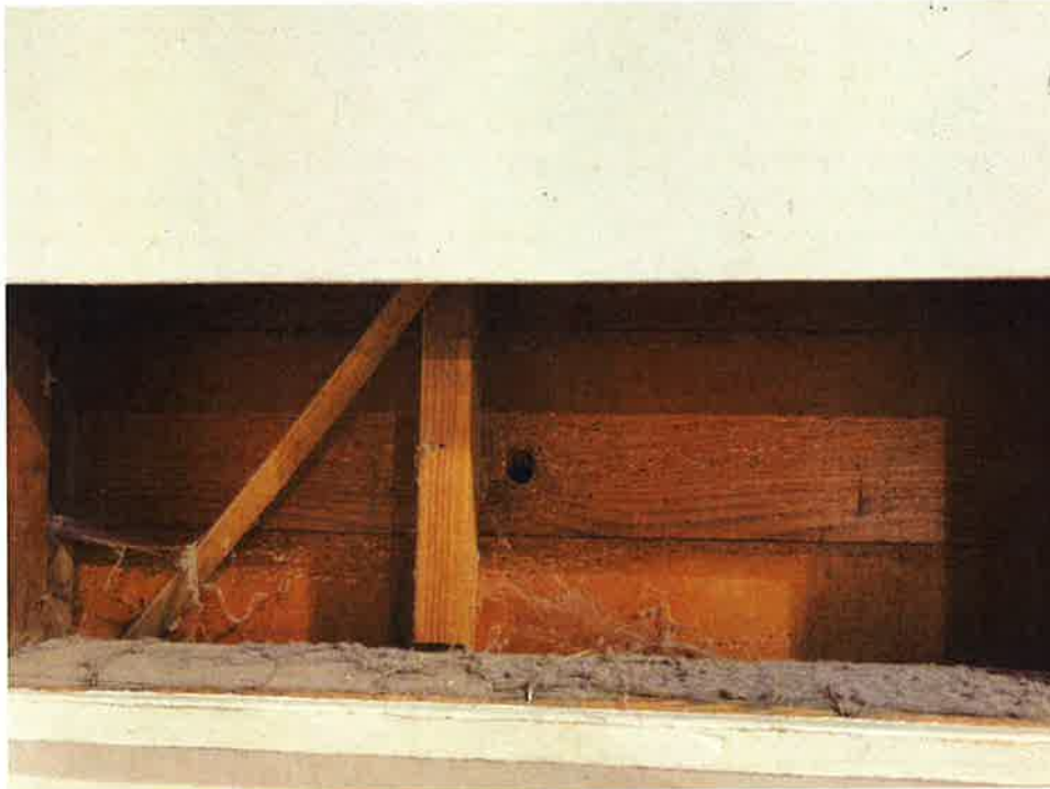
Figure 7: Wall Farming – Wall studs w/ exteriors 1x decking as sheathing
