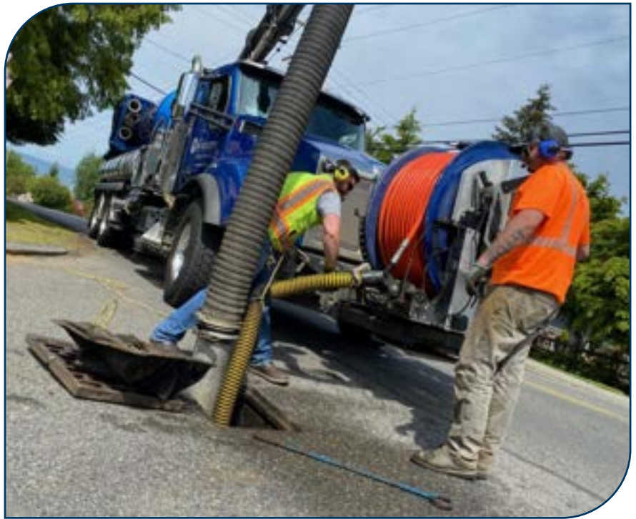
Cleaning pipes in advance of CCTV inspection.
