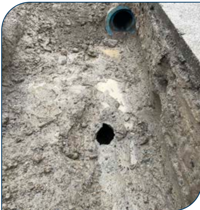
Broken stormwater pipe.
