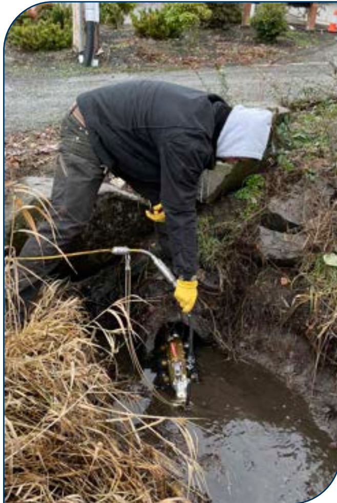
Using camera to inspect culvert connected to open channel conveyance.
