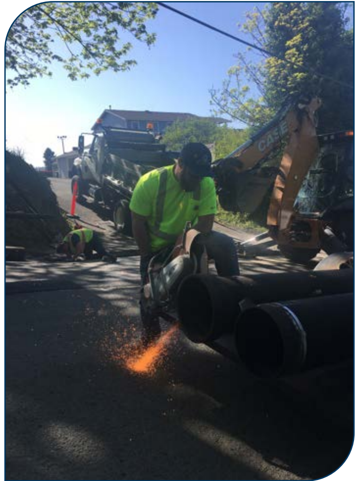
Cutting pipe for a pipe replacement project.
