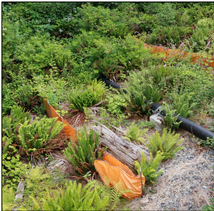
Stormwater Outfall Pipe on Slope (HDPE Smooth Pipe)
