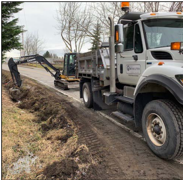
Storm Crews Conducting Open Channel (Ditch) Maintenance.
