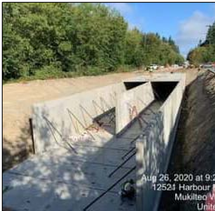
Stormwater Vault on Harbour Reach Dr., Mukilteo.
