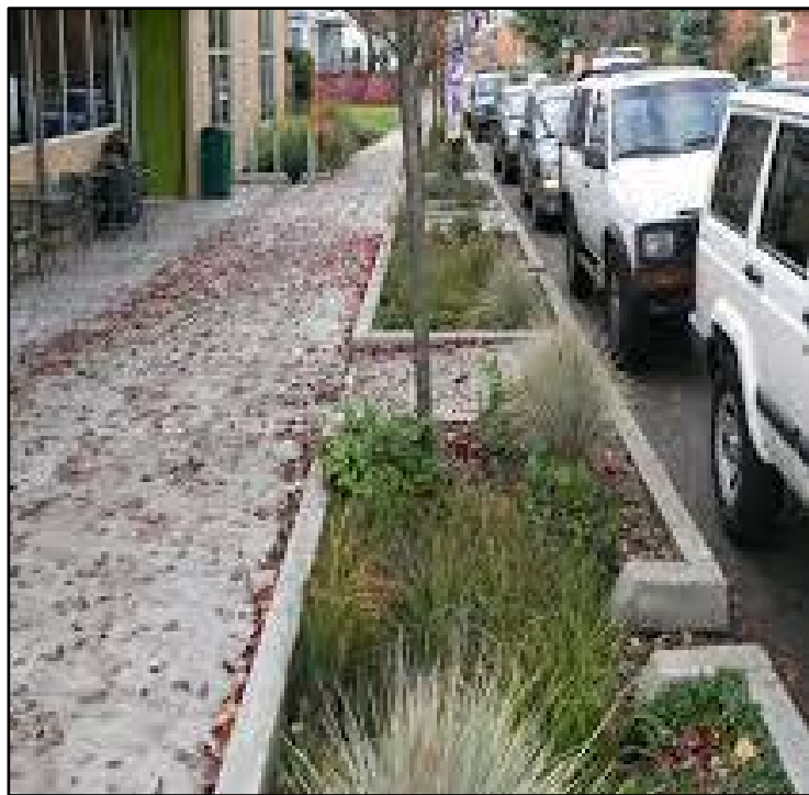
Bioretention swale photo. From Washington Stormwater Center.
