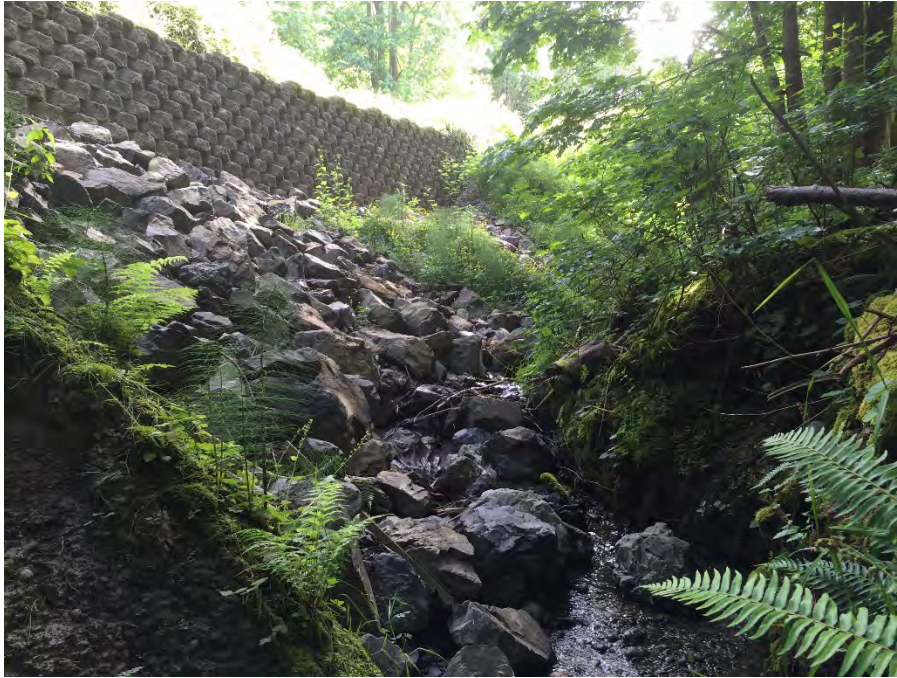
Photo #6. Concrete block and rip rap slope stabilization on right bank.
