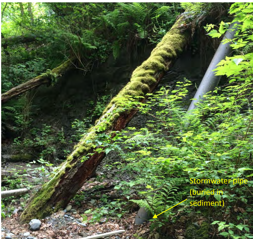
Photo #4. Twelve-inch diameter solid wall polyethylene pipe (tightline) buried in sediment and debris.
