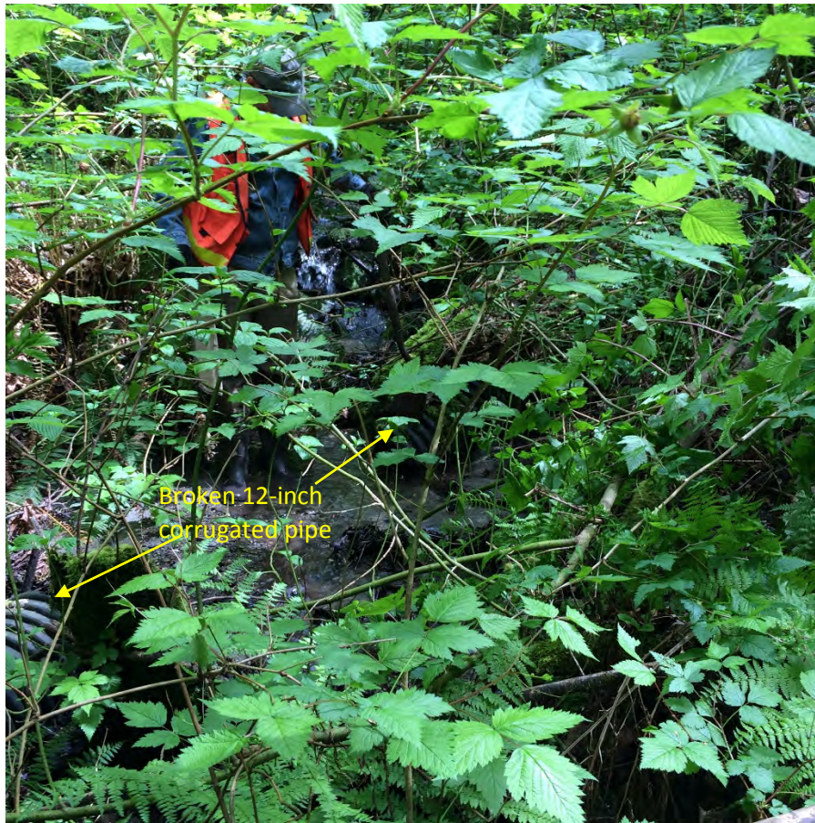
Photo #11. Broken tightline (12" corrugated black plastic) originating from left bank.
