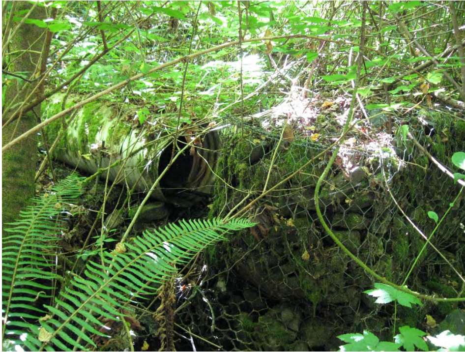
Photo #8. Left bank 18-inch-diameter corrugated metal pipe with gabion outfall energy dissipation structure. Pipe is lined with interior plastic pipe.
