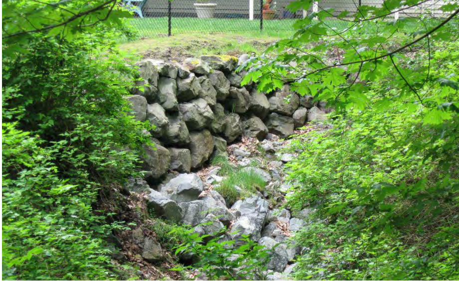
Photo #13. Right bank slope stabilization with rip-rap.
