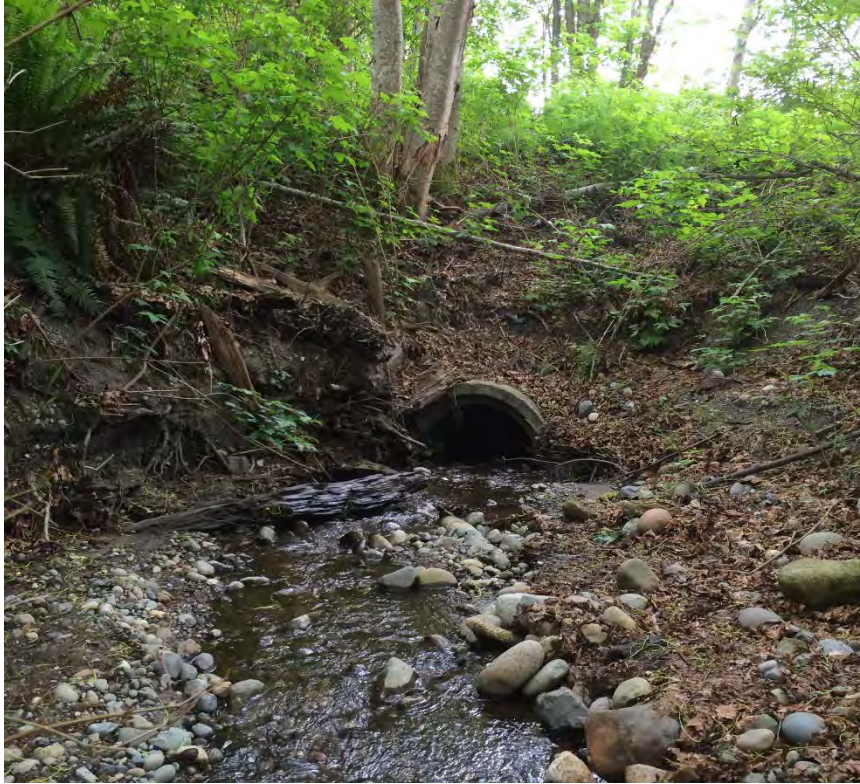
Photo #15. Upstream end of 3-ft diameter concrete culvert.
