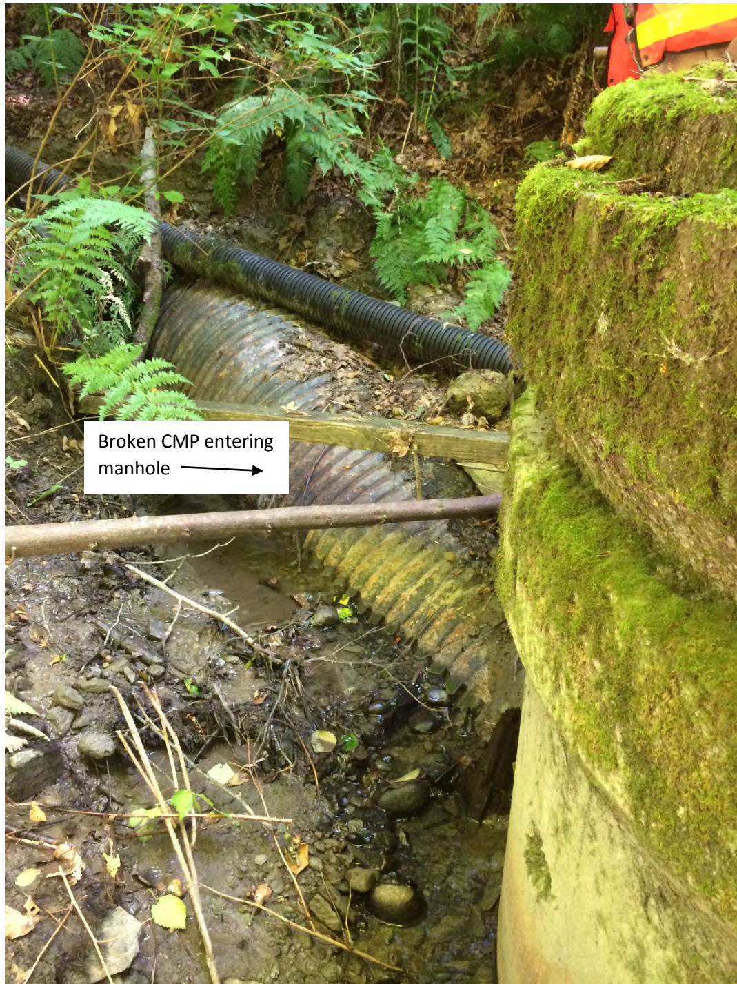
Photo #5. Upslope on right bank from CMP outfall. Pipe entering manhole is broken and flow is going around manhole and eroding slope. Small diameter black drainpipe is also being used to route flow from upslope.
