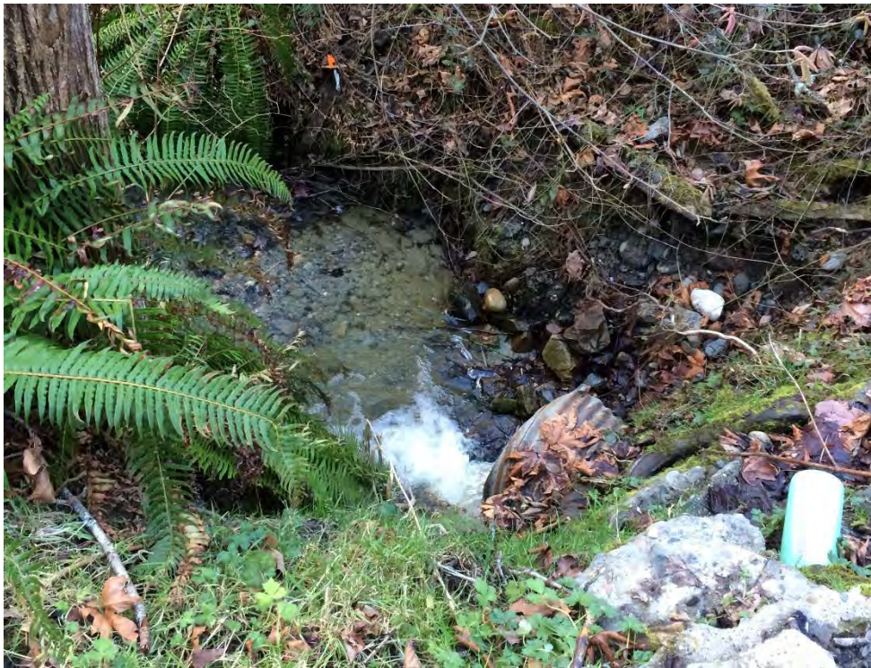
Photo #9. Culvert (24-in-diameter corrugated metal pipe) crossing under 61 st Place SW. Culvert is perched 2 feet above the channel bed.
