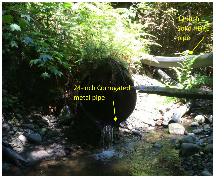
Photo #4. 24-inch corrugated metal pipe entering channel from right bank. Note HDPE has sag due to erosion of stream bed and hillslope on the left side of the photo.
