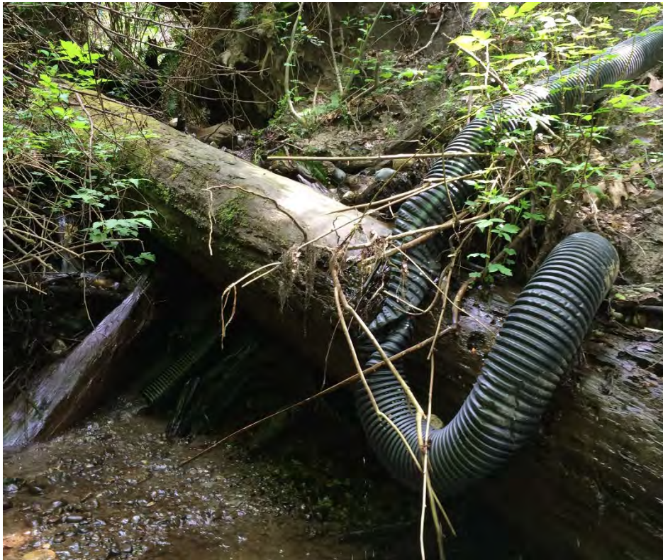
Photo #6. Example of damaged drain pipe in channel (many broken pipes were observed).
