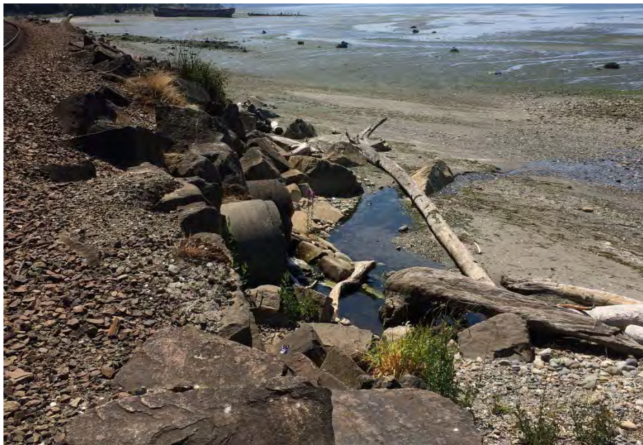
Photo #1. Looking south at two 42-inch concrete culverts at low tide.
