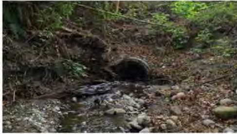
Upstream end of culvert under maintenance road.
