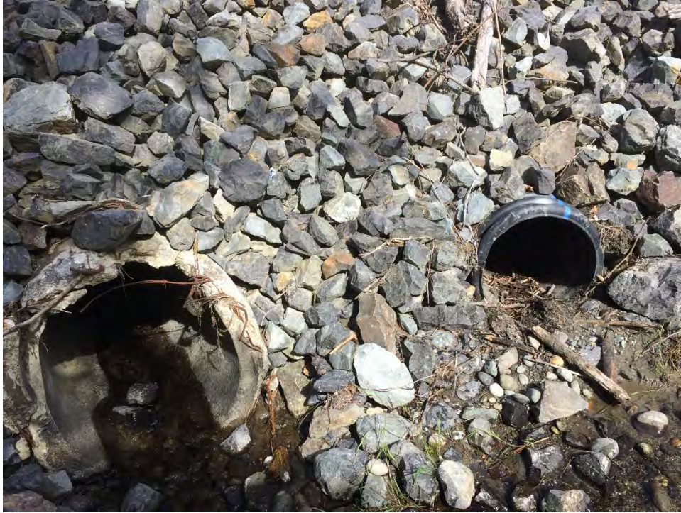
Photo #2. Upstream end of Smuggler's Gulch creek outfalls (30-in-diameter concrete culvert on right of photo and 18-in corrugated plastic culvert on left of photo).
