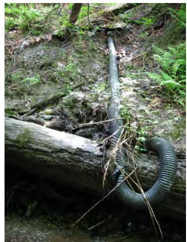
Photo 2. Example of mangled drain pipe
