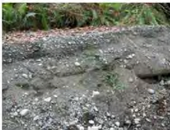
Sediment deposition upstream of maintenance road culvert.
