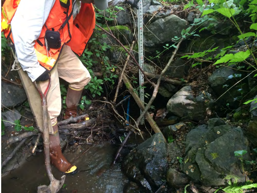
Photo #4. Squashed corrugated metal culvert under private driveway. Photo is from upstream end.
