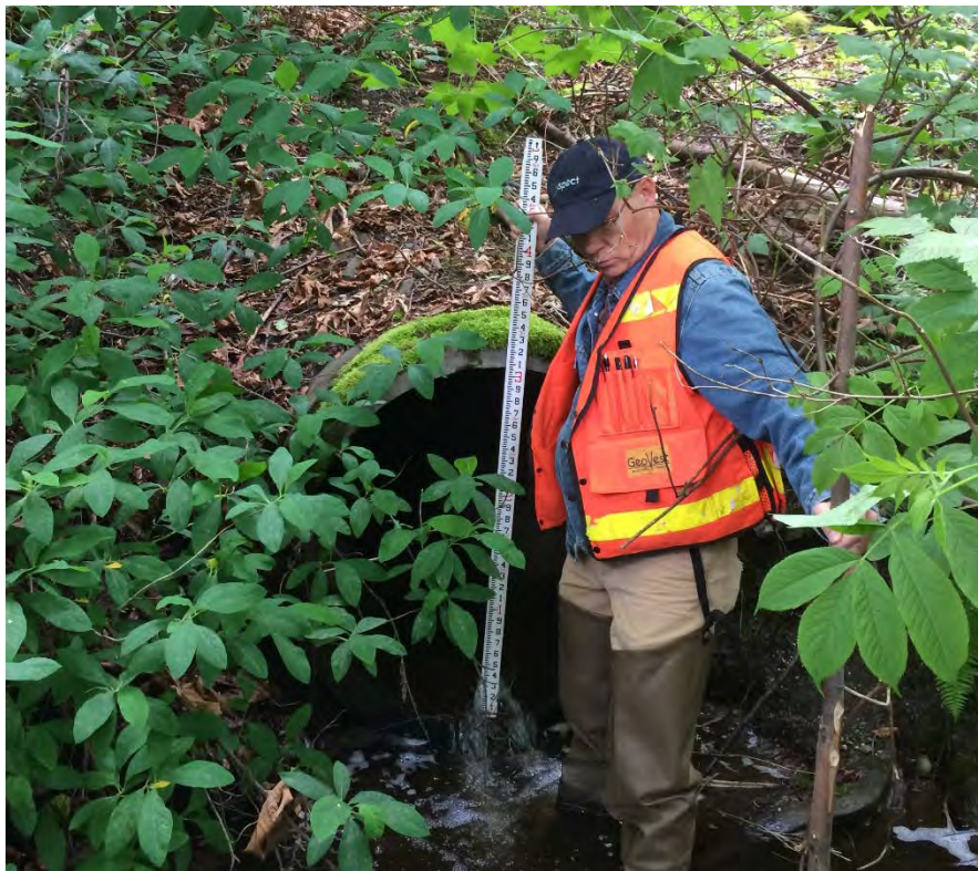
Photo #14. Downstream end of 3-ft diameter concrete culvert under access road.
