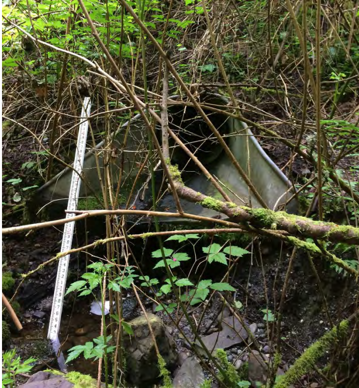
Photo #23. 18-inch corrugated metal culvert on right bank (broken).
