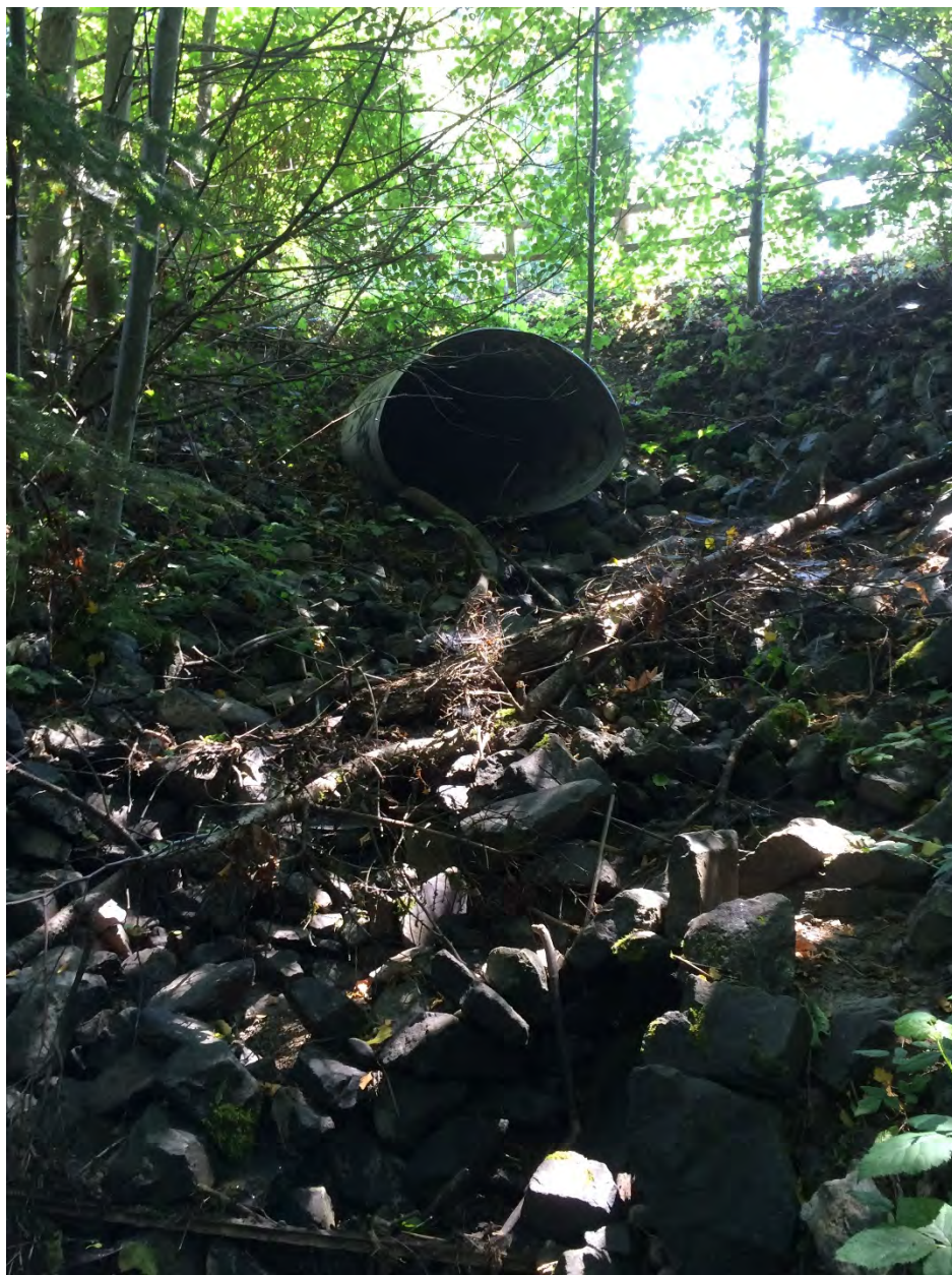
Photo #18. Squashed corrugated metal culvert under Surrey Lane.
