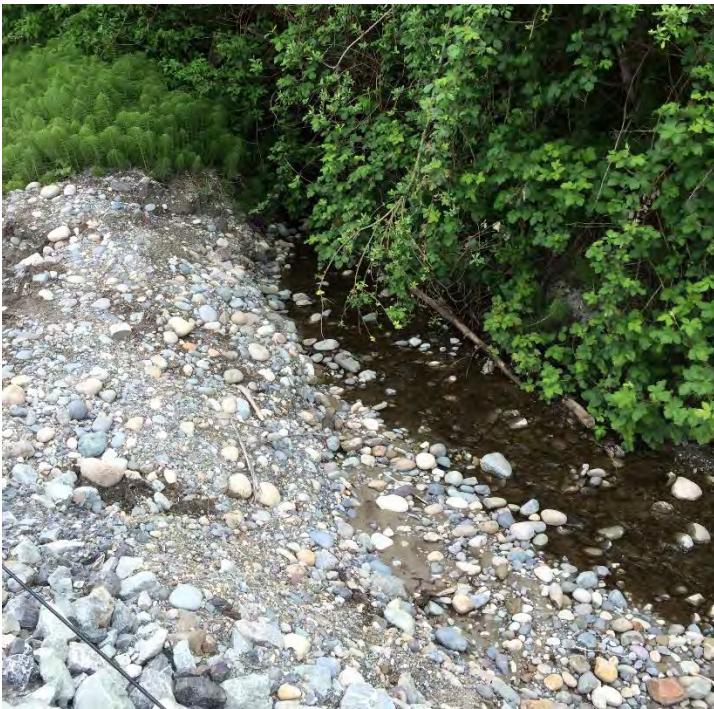
Photo #2. Sediment accumulation on upstream side of culvert under BNSF railroad tracks. Cobble sizes range from 3 inches to 8 inches in diameter.
