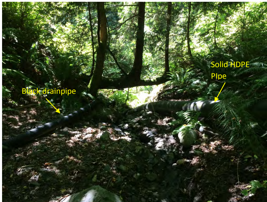
Photo #6. Downslope from manhole. Black drainpipe on left of photo and 12-inch HDPE on right.
