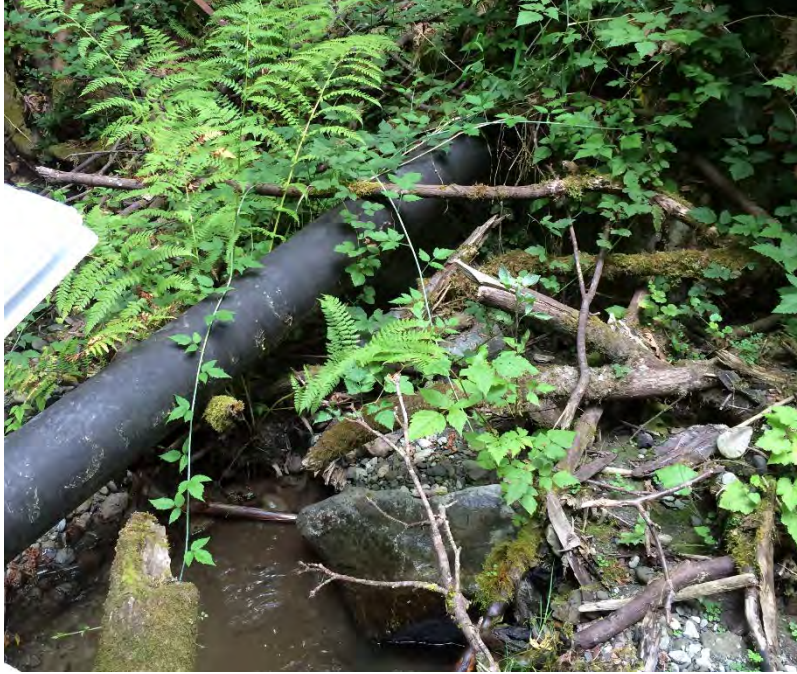
Photo #8. Solid wall pipe on left bank.
