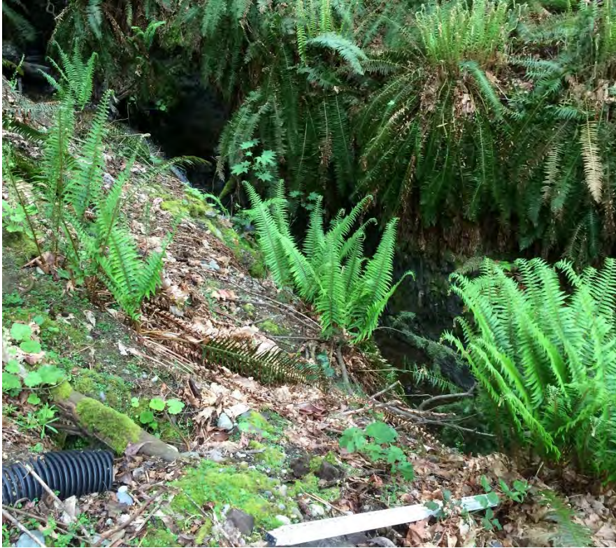
Photo #11. Right bank broken drain pipe and T-section. Channel is incised about 8 feet in this location.
