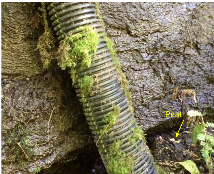
Photo #13. Left bank drainpipe with pre-Fraser non-glacial deposit with erosion resistant hard peat layers in background.
