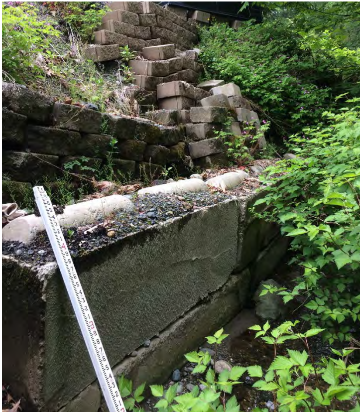
Photo #20. Concrete block revetment on right bank.
