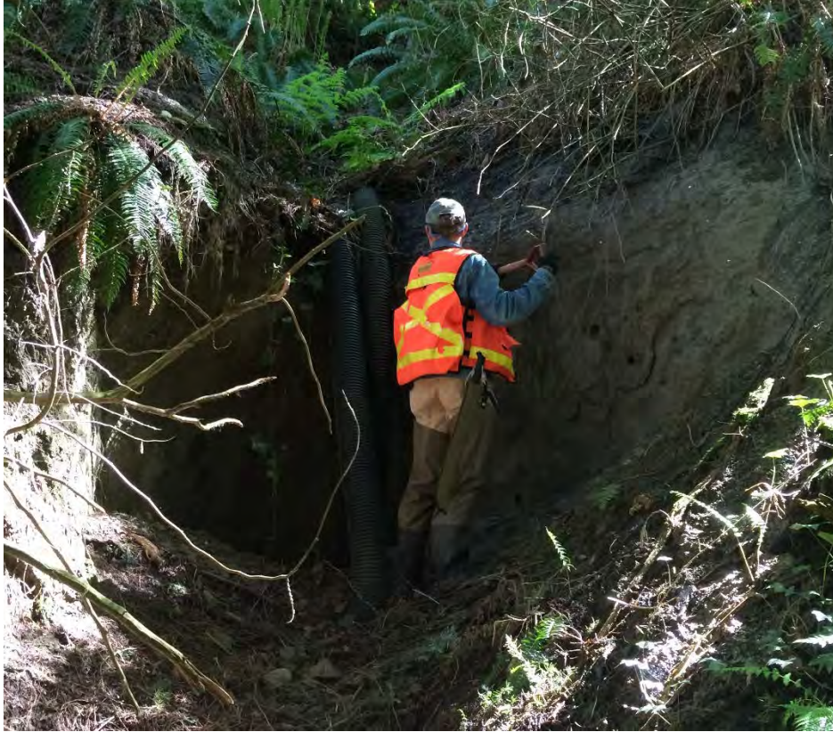
Photo #7. Broken tightline and eroded gully on right bank approximately 50 feet east of channel.
