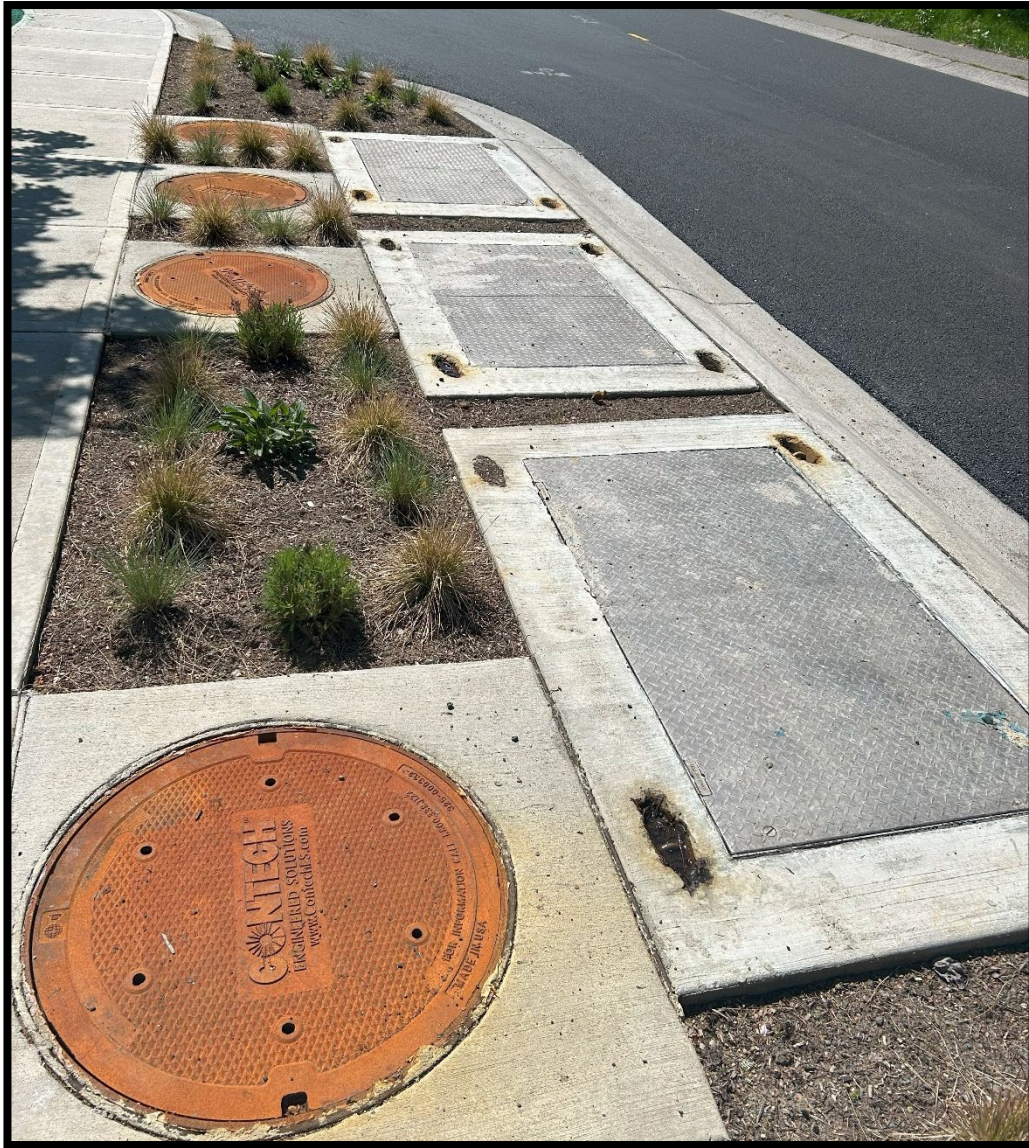
New low-impact development water quality structures were installed at 47th Place W in early 2025.
