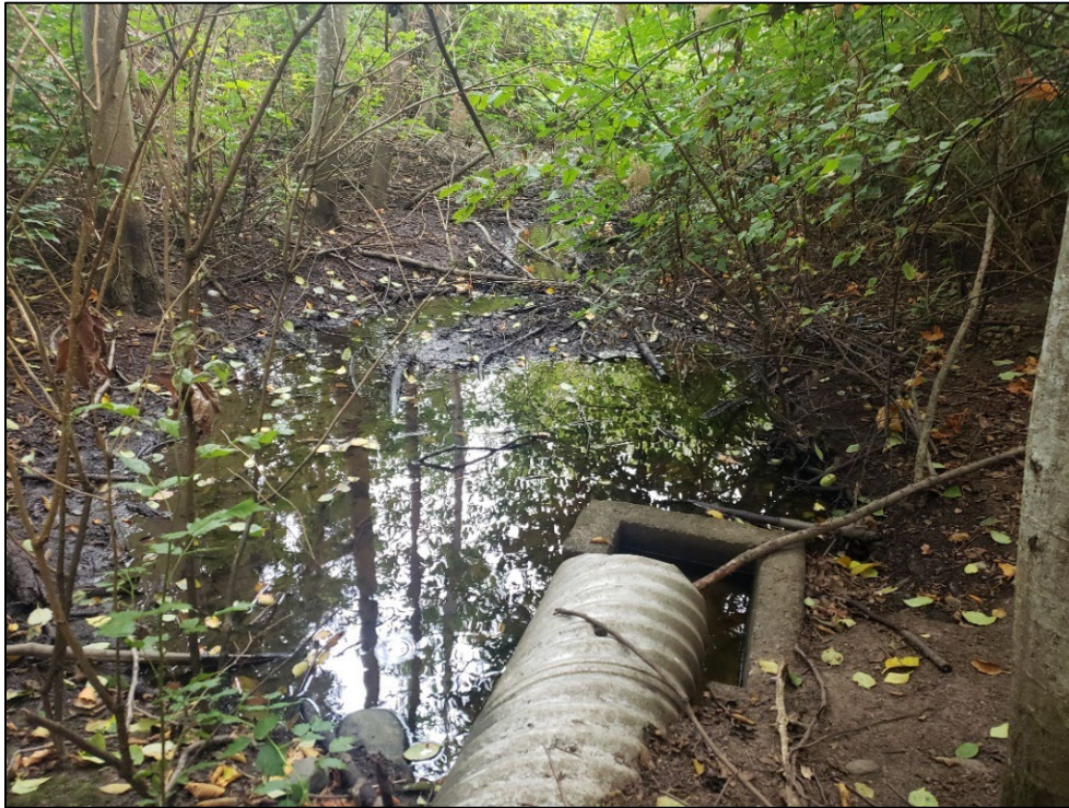
Photo 1. Inlet to stormwater feature via an 18" metal corrugated culvert.
