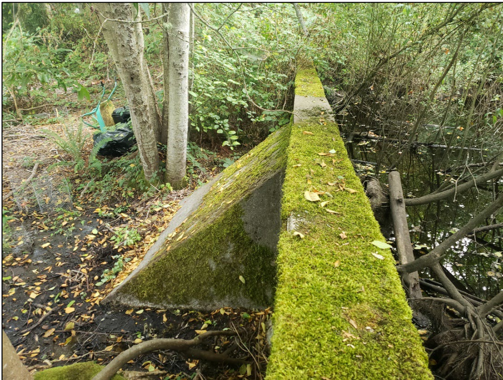
Photo 4. Seepage occurring downslope of the retaining wall and spillway structure, saturated soils noted on left.
