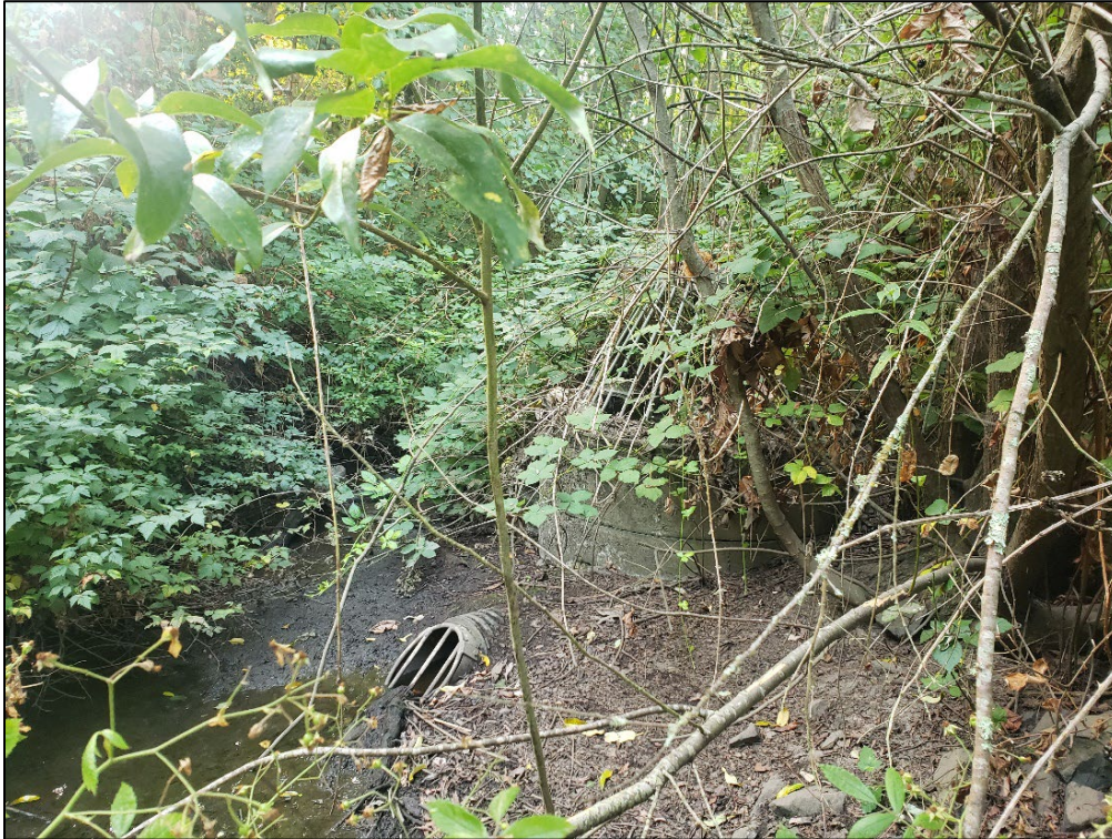
Photo 3. Stormwater feature outlet and overflow structure with bird cage.
