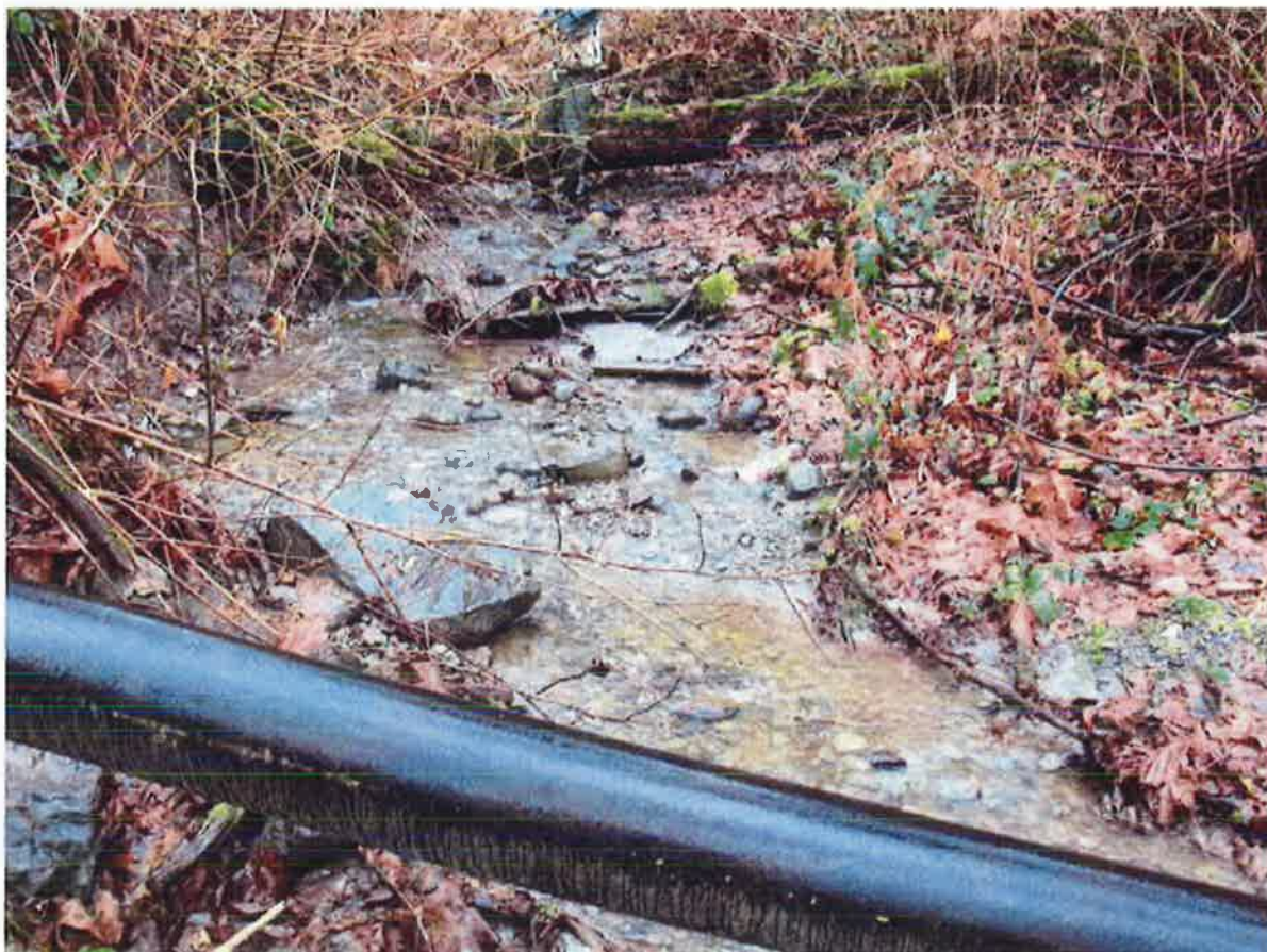
Photo 2: Stream channel with exposed sewer pipe crossing stream in foreground, indicative of historic downcutting and channel incision
